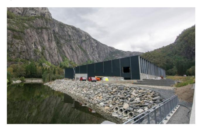
The freshwater plant at Fjæra in Norway was completed in 2018, combining a high-quality freshwater source with state-of-the-art recirculating aquaculture systems (RAS) so as to control and maximise smolt production while minimising freshwater usage.
