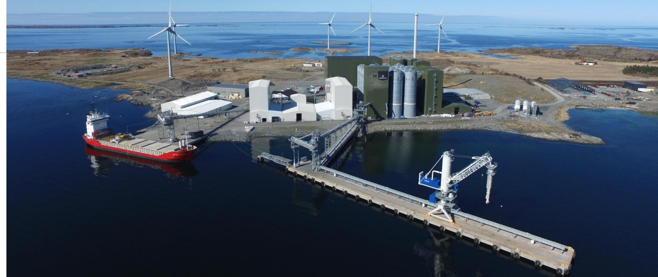
Scotland: New plant
